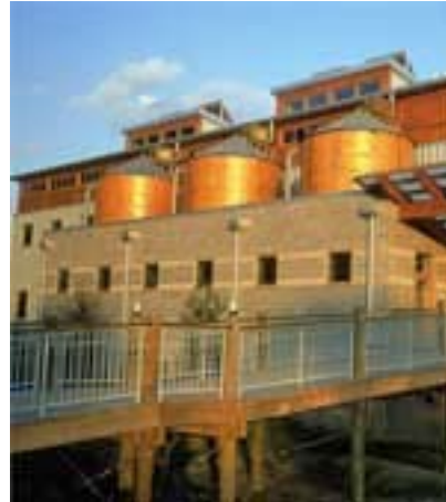
Three cisterns atop the Phillip Merrill Environmental Center Courtesy of the US Dept. of Energy
