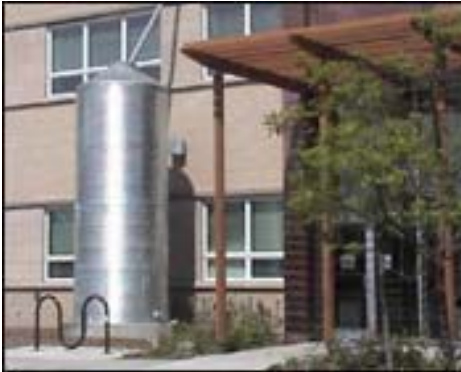
One of four 12,000 gallon cisterns at Chicago Green Tech Headquarters Photo courtesy of Chicago Green Tech
